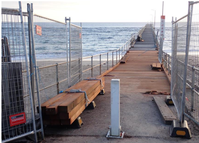
Repairs to Port Noarlunga Jetty underway! Photo courtesy of Alex Suslin
