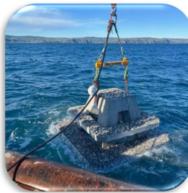
One of the modules being placed into position.
